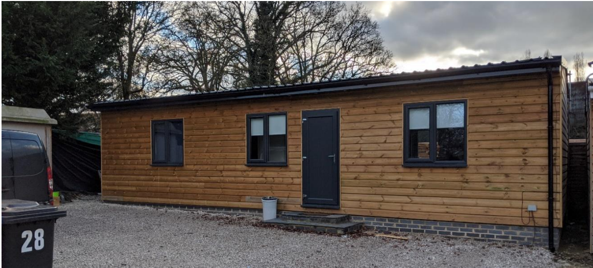
Figure 2- Existing building on site.
