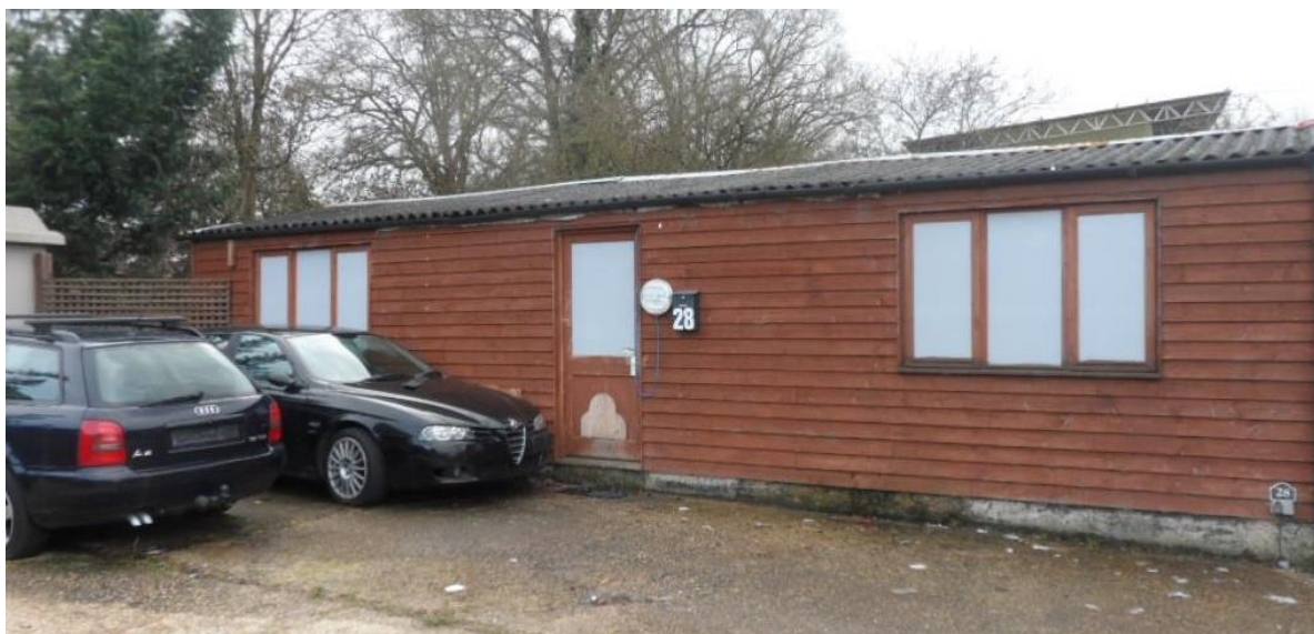
Figure 1 -Subject building May 2016
